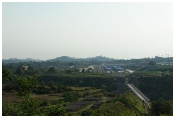
Picture 6-7: Railway line
