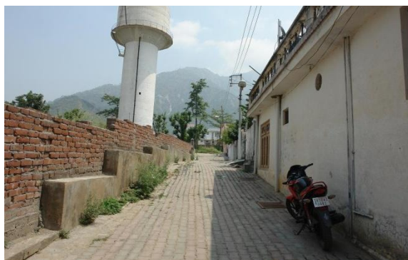
Picture 5-1: Overhead water tank
